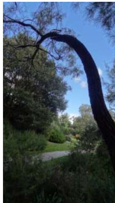
Figure 8. Tree 95 – heavy lean over footpath
